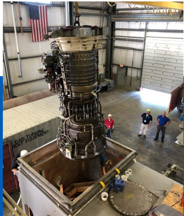
Engine removal and maintenance verification
